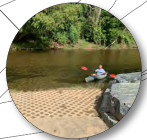
Decking platform or kayak launch point
